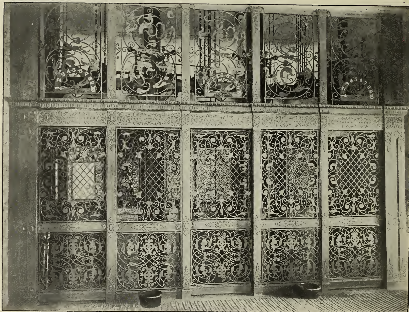
ELEVATOR INCLOSURES, MAIN FLOOR, TEUTONIC BUILDING, CHICAGO.
